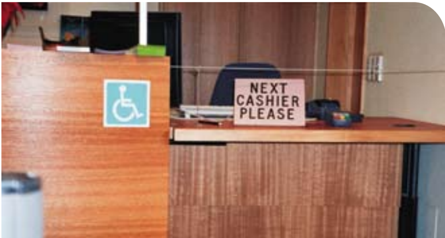
An accessible counter that is not used because the cashier operates from another part of the counter.
