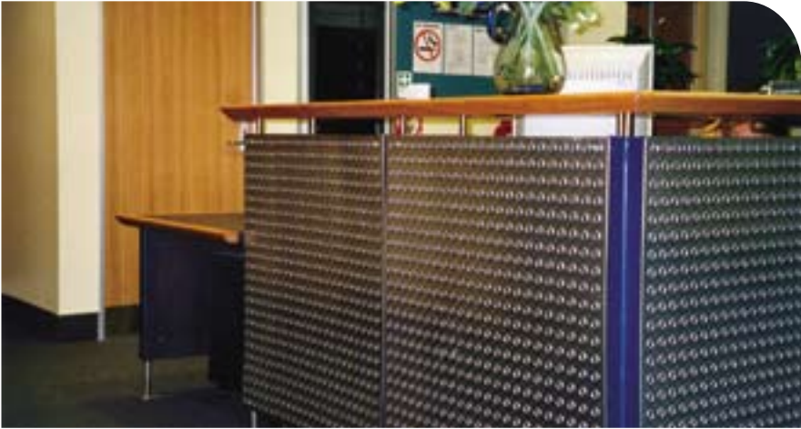
A high reception counter with the accessible section around the corner and not visible on entering.
